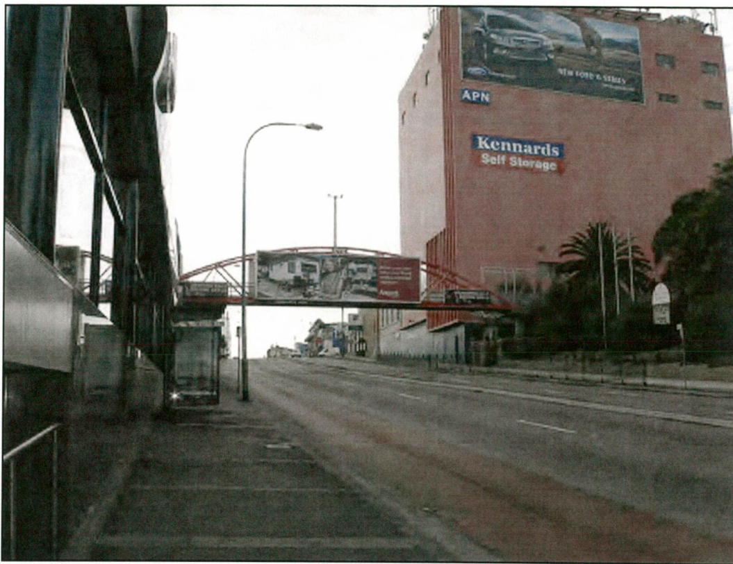
Photograph 1: View east to the subject site from northern footpath.
