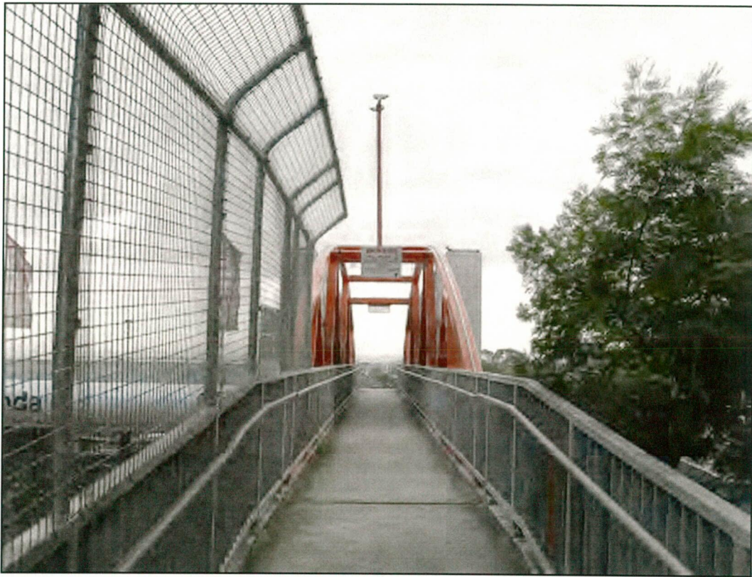
Photograph 5: View north across the pedestrian bridge.
