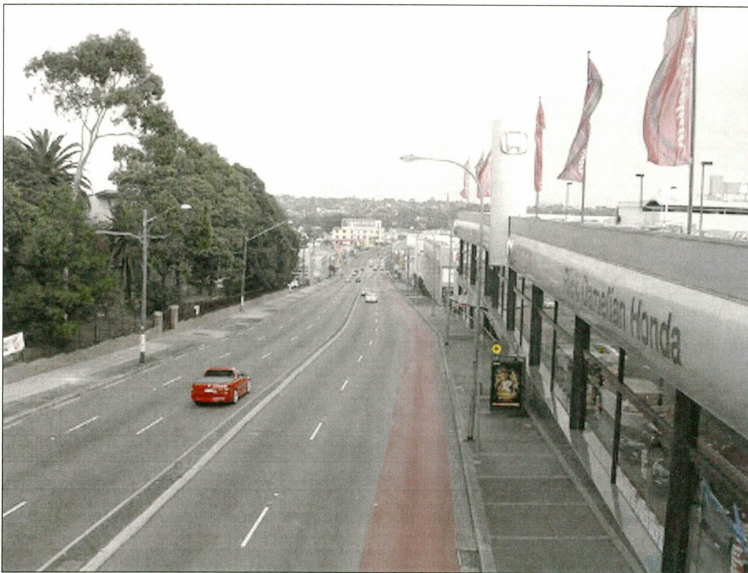
Figure 2-3 View west from the existing pedestrian bridge
