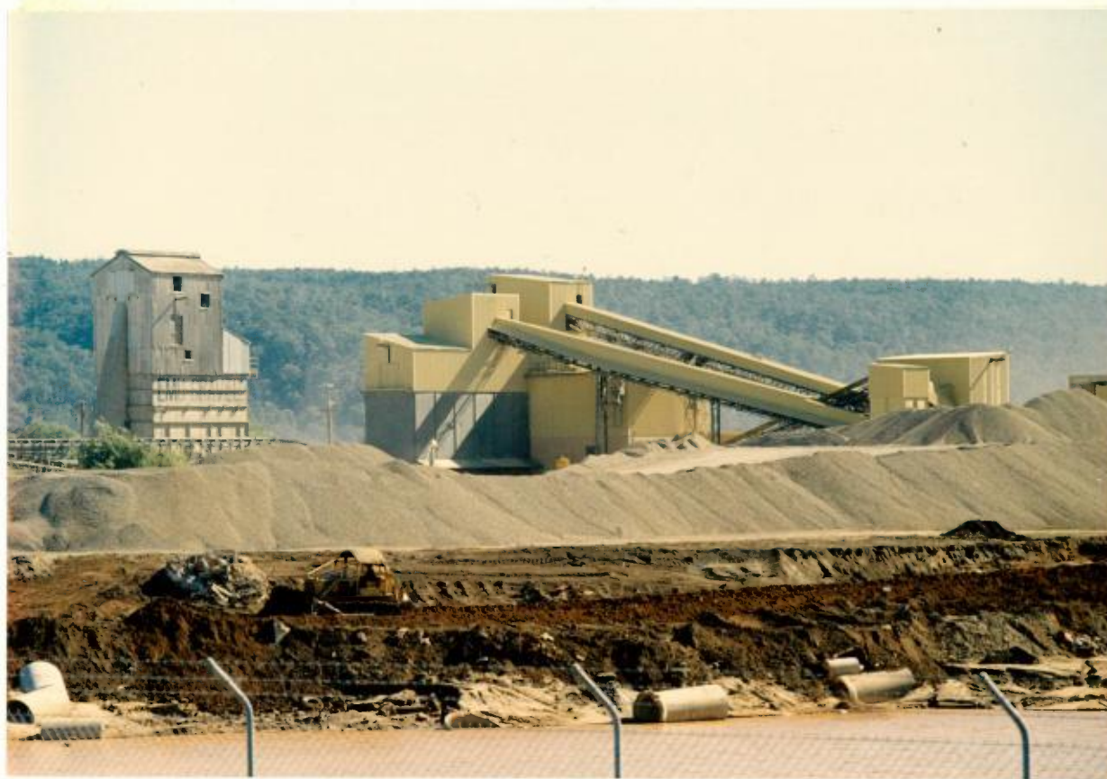
PLATE 1: Old and New Processing Plants, Product Stockpiles and Pit Backfilling.
