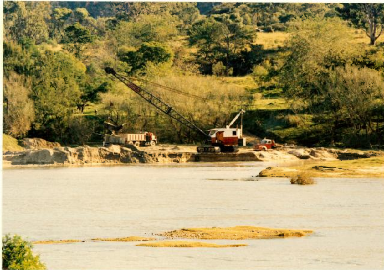
PLATE 8 : Underwater River Gravels being excavated by Dragline and Trucks.
