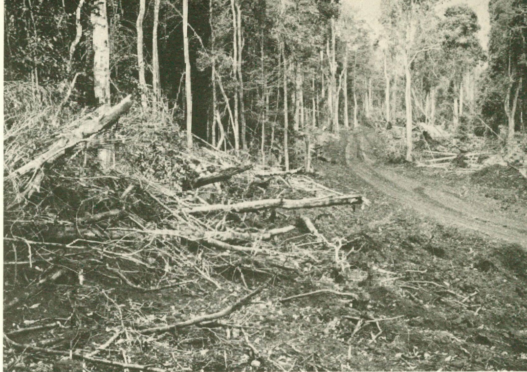
Forest access road and logging operation, Cangj State Forest
