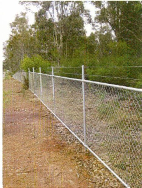
(B) 6-ft chain mesh fence ($30-40/m)
