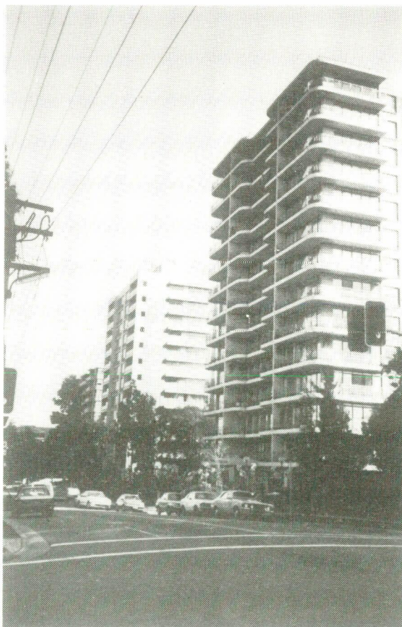
Good distance separation, as illustrated in these examples, is the main means of ensuring an acceptable degree of privacy in multi-storey developments
