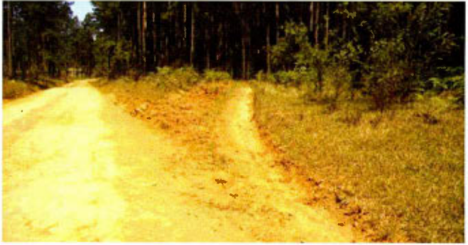
Figure 5.9: Mitre drain
