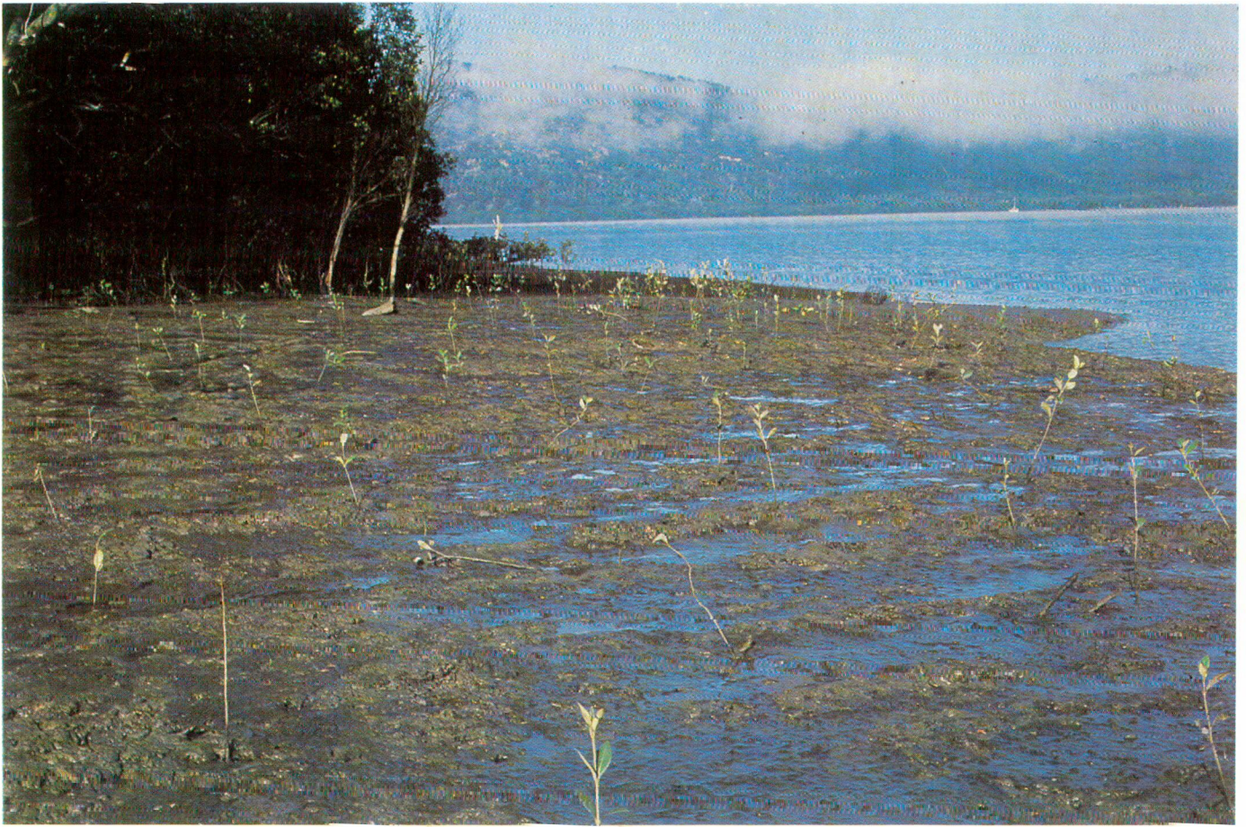
Foreshore-restoration works at the Hawkesbury River
