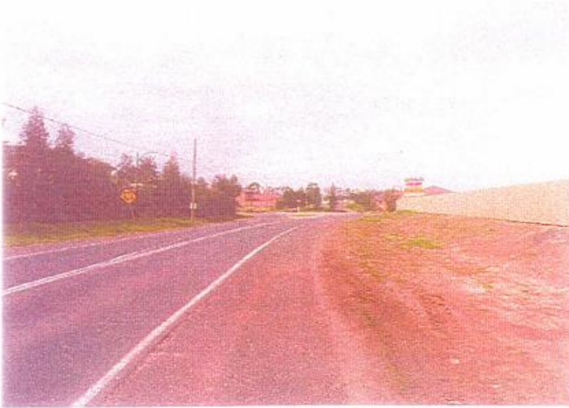
Figure 3.1: View to north along Beech Road through modern housing estate. This road will be widened to 4/5 lanes. Modification 1. 1 August 2001.
