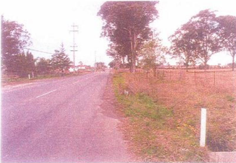
Figure 3.2: View to south along Bernera Road, Prestons. The road will be widened along the western side where a strip of land will be acquired. Modification 3. 1 August 2001.
