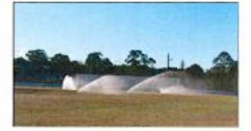
EXISTING IRRIGATION SYSTEM
