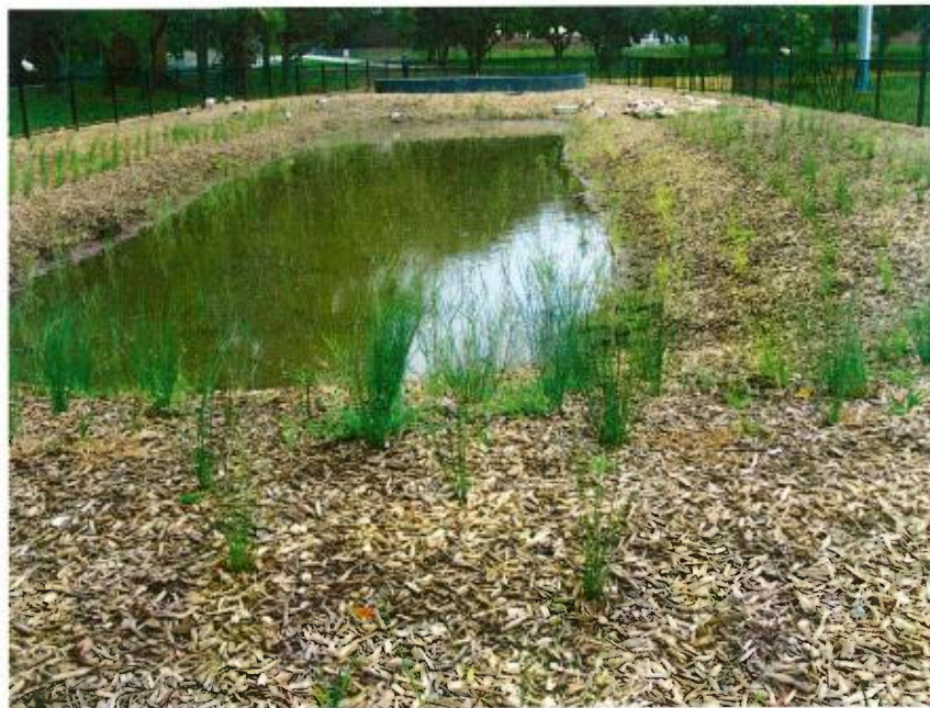
Mackey Park Wetland – sports fields storage and drainage treatment system, December 2010.
