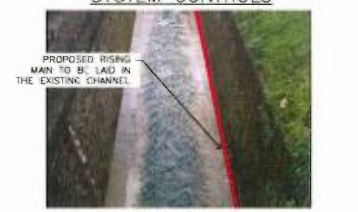
EXISTING STORMWATER CHANNEL
