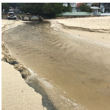
Stormwater drain flow
