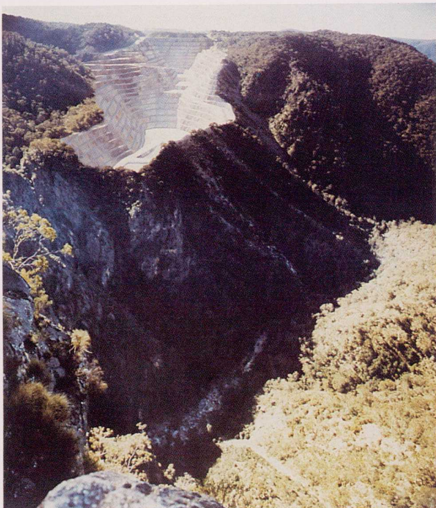
Marulan Quarry — Phase 2
