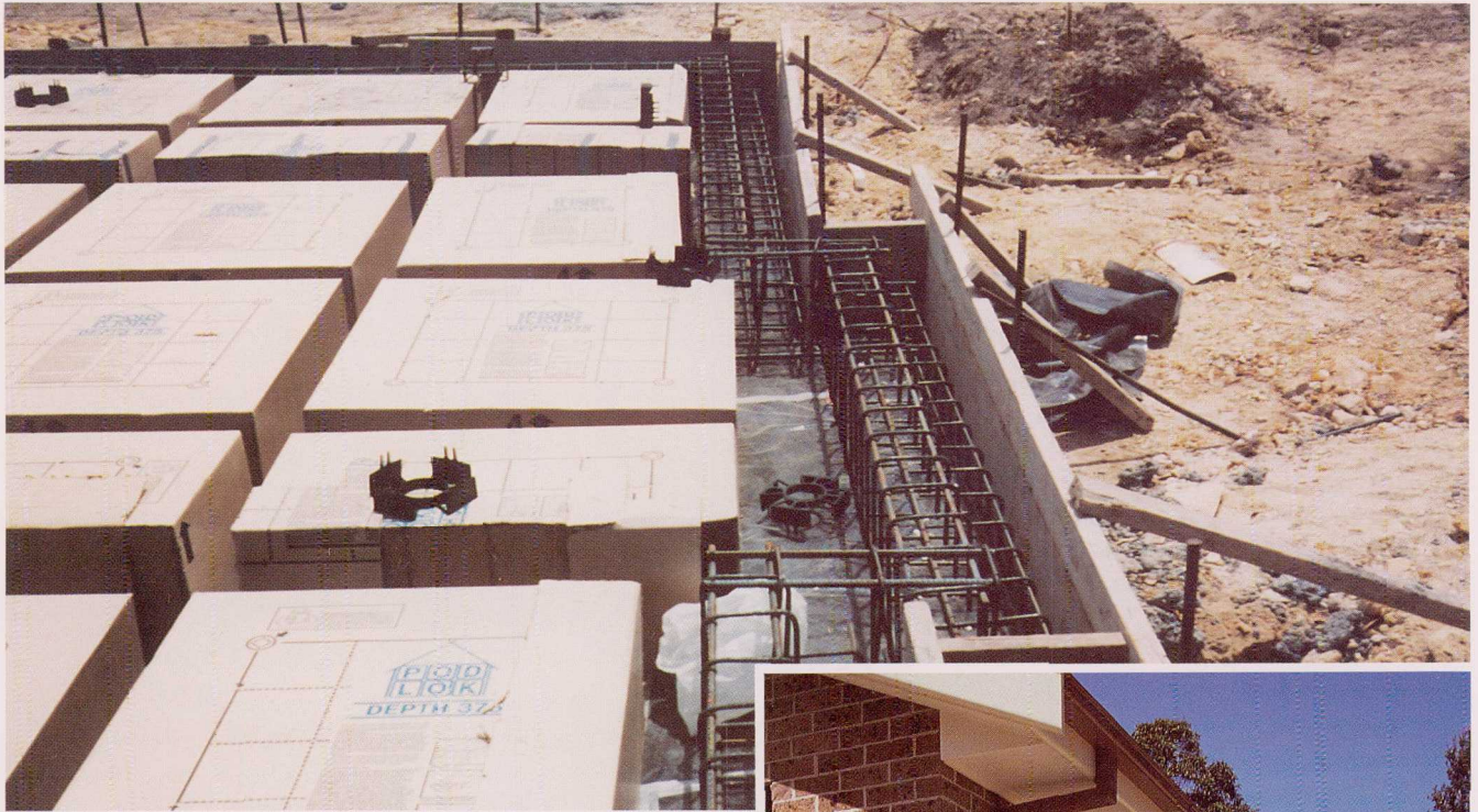
Above: The waffle raft slab before pouring concrete for test house at Wyee State mine
