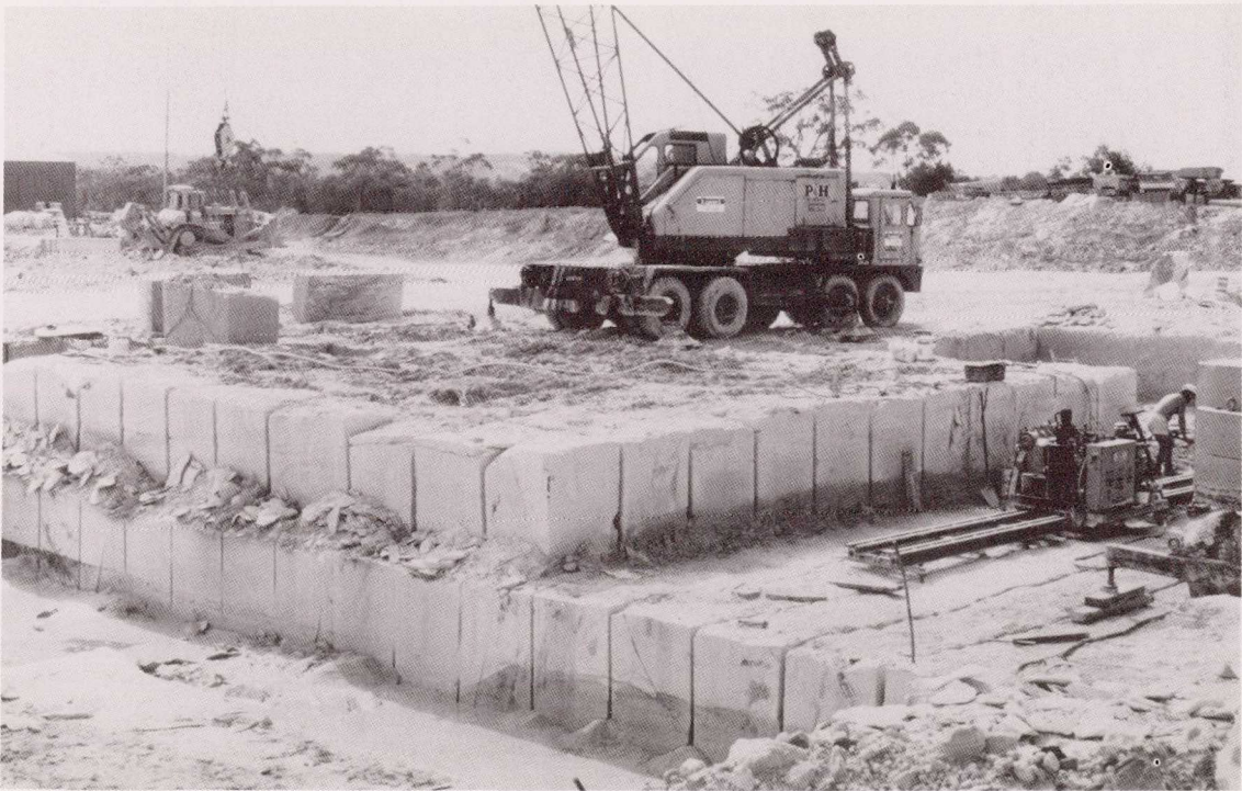
Quarry block being lifted at Central Coast Sawn Stone Quarries' Somersby quarry. Note the channel configuration and the Korfmann saw on rails (right)
