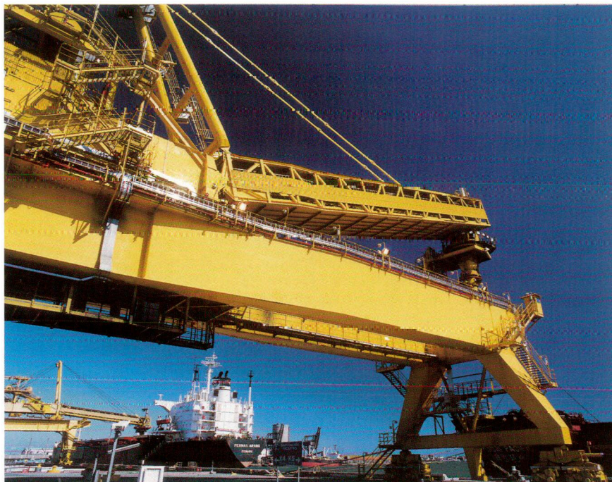
The new coal ship loader at Kooragang Island near Newcastle. In the background the first loader can be seen loading coal for export to Korea
