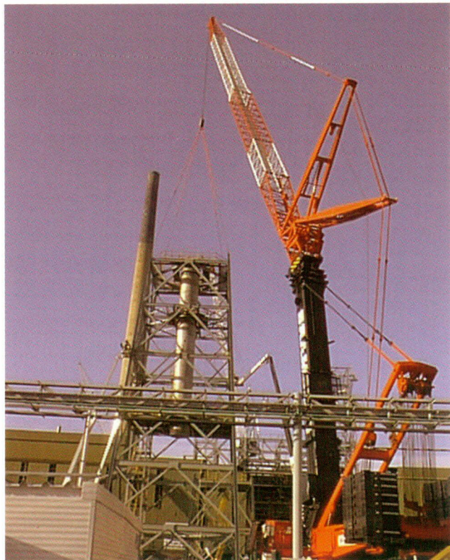
Acid stack under construction
