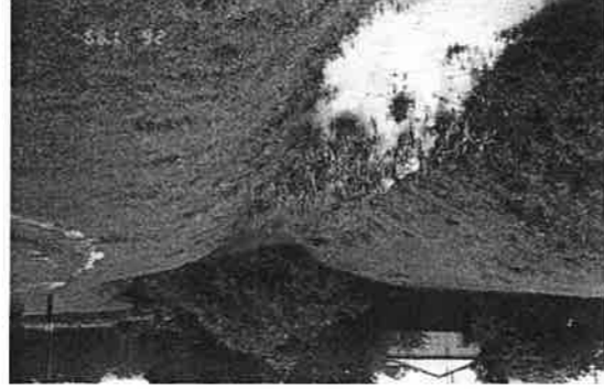
42. Stormwater channel runs into underground drain - erosion and weeds are issues here
