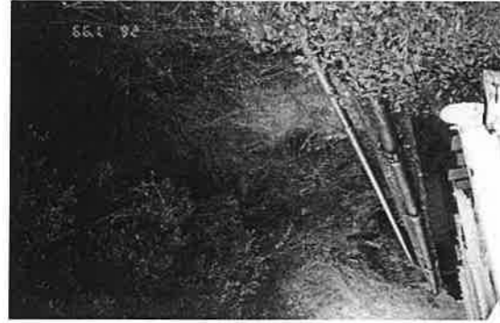
42. Stormwater channel runs into underground drain - erosion and weeds are issues here
