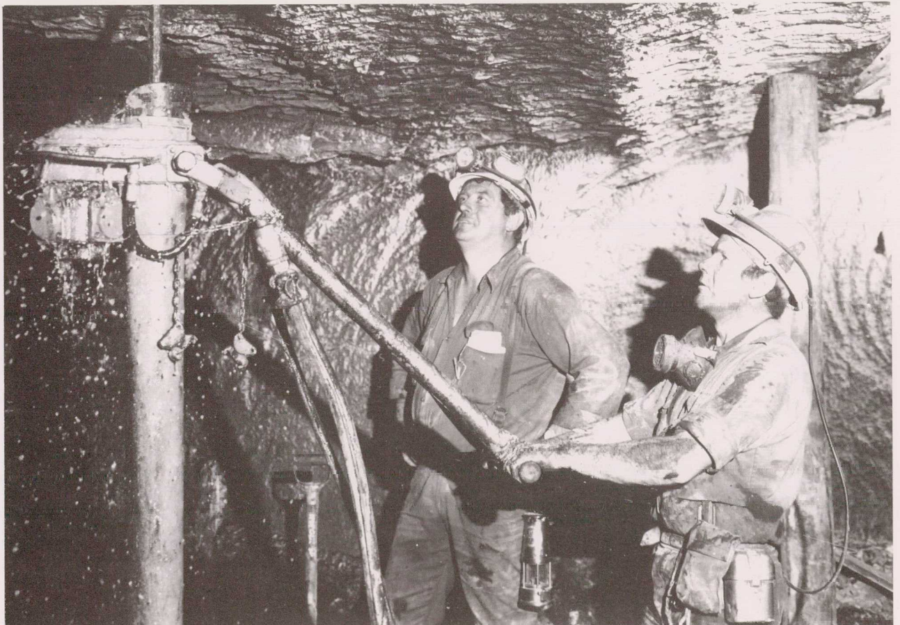
Roofbolting, Newvale colliery
