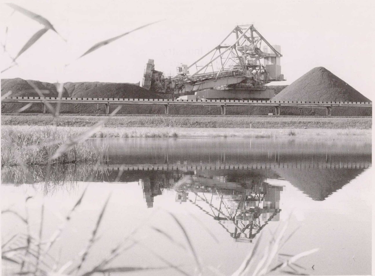
Coal stacking area, KCL coal loader
