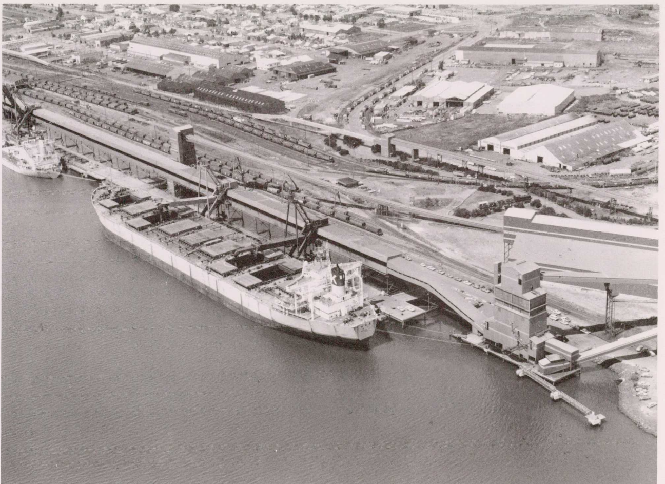
Shiplading berths, PWCS coal loader
